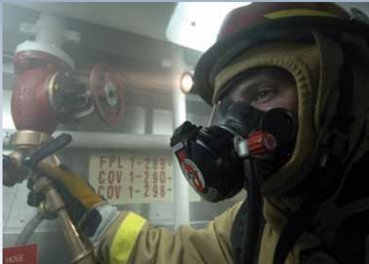
Straight & Angled Hose Globe Valves IAW Navy DWG 1385711/12
