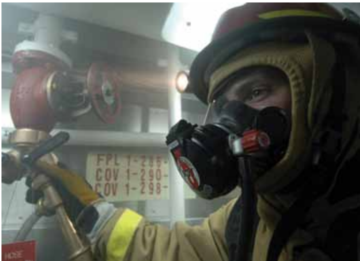
Straight & Angled Hose Globe Valves IAW Navy DWG 1385711/12
